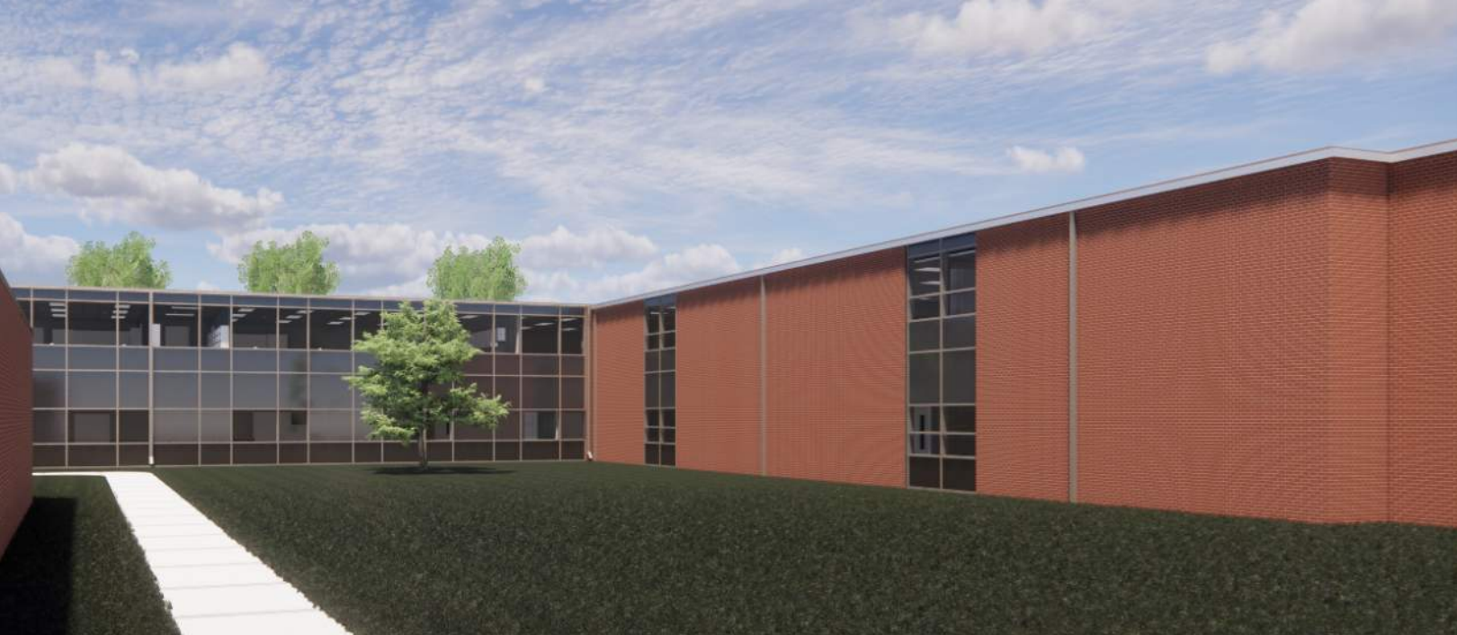
EXTERIOR VIEW OF NEW CURTAINWALL
