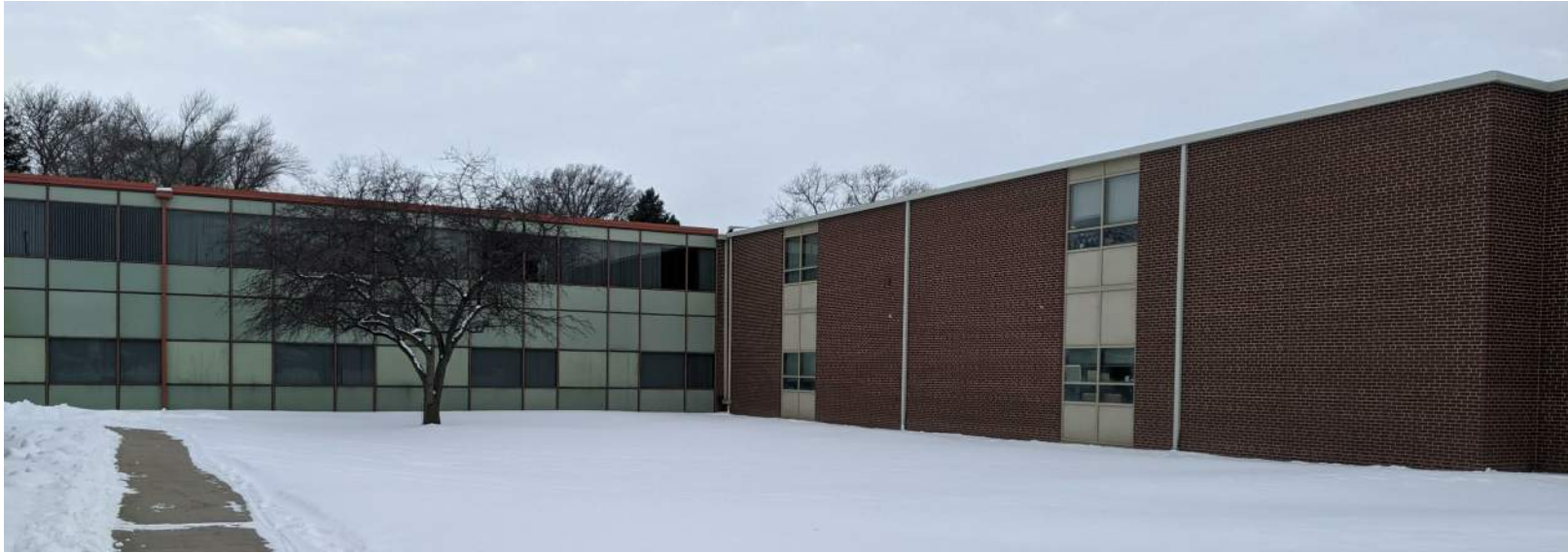
EXTERIOR VIEW OF EXISTING CURTAINWALL
