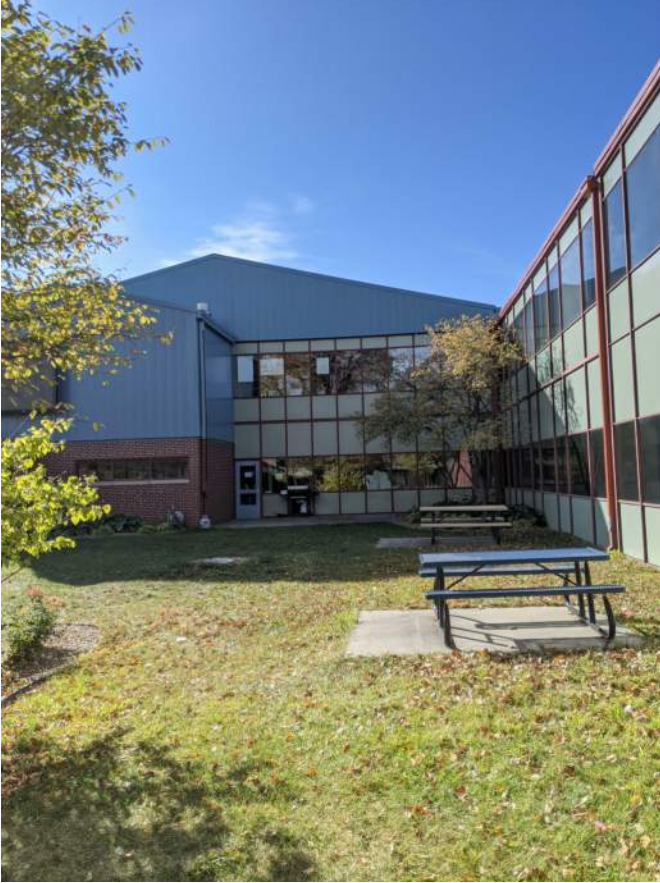
EXTERIOR VIEW OF EXISTING CURTAINWALL
