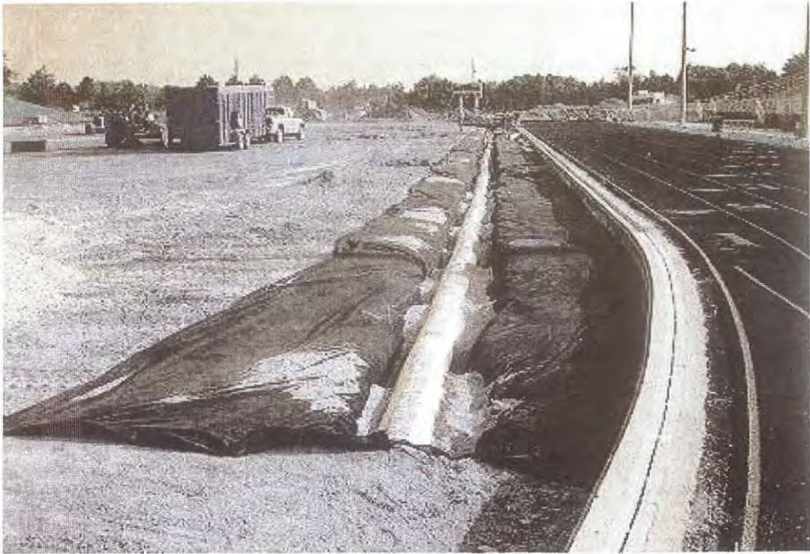
Drain at perimeter of playing field
