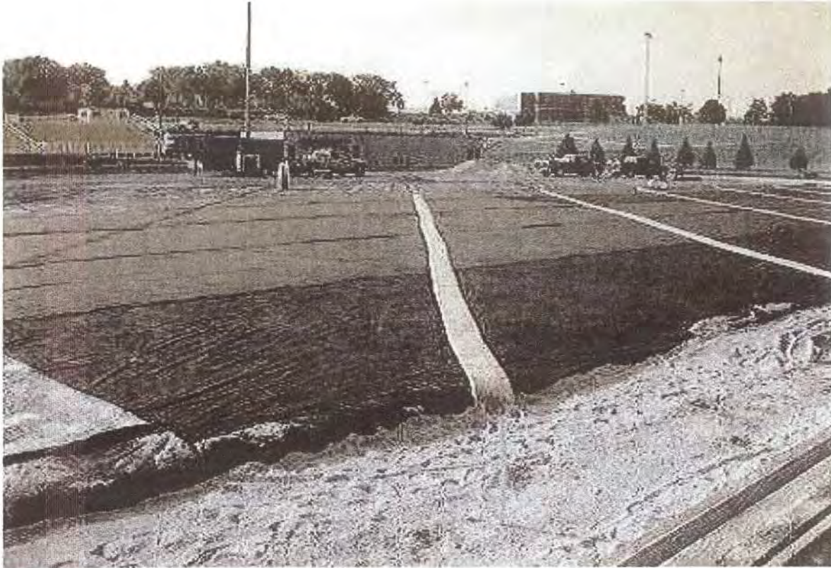
Lateral Drains in playing field area
