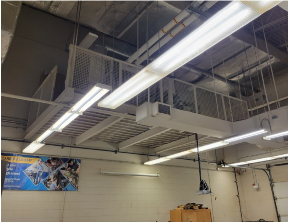
Figure 2 - AHU serving construction tech classrooms
