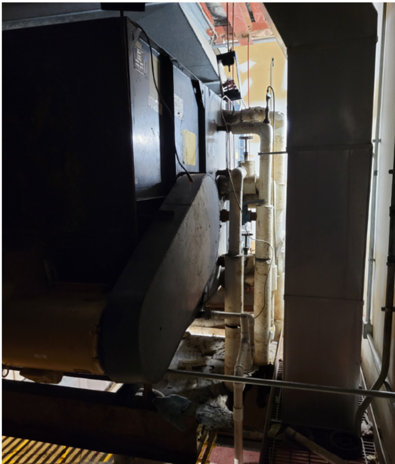
Figure 3 - AHU Serving Competition Gym and Wrestling Room
