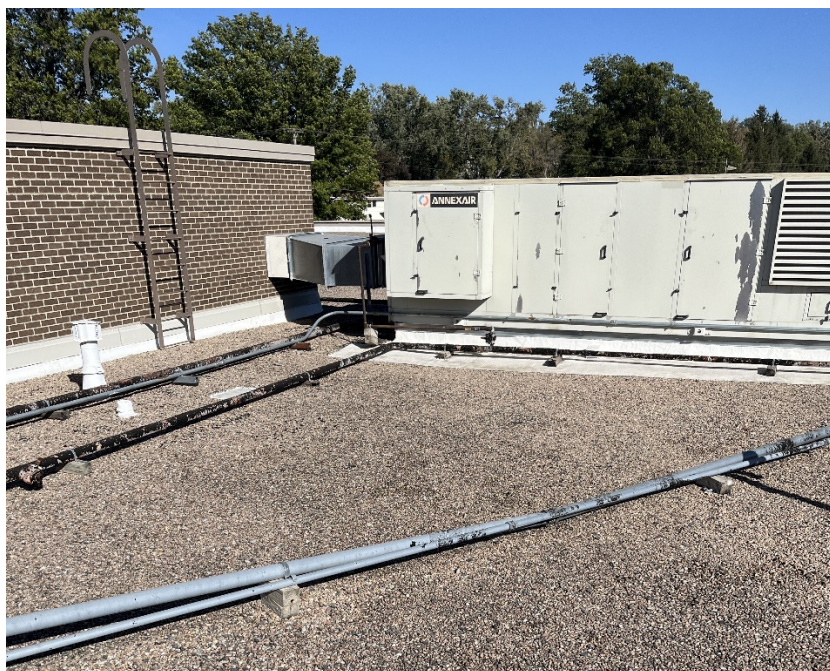
Existing Multizone RTU
